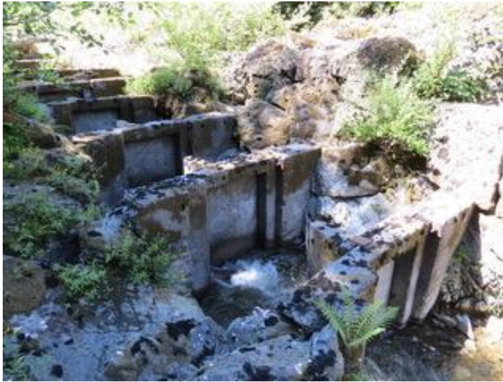
Figure 51. Fish way constructed to improve fish habitat.
